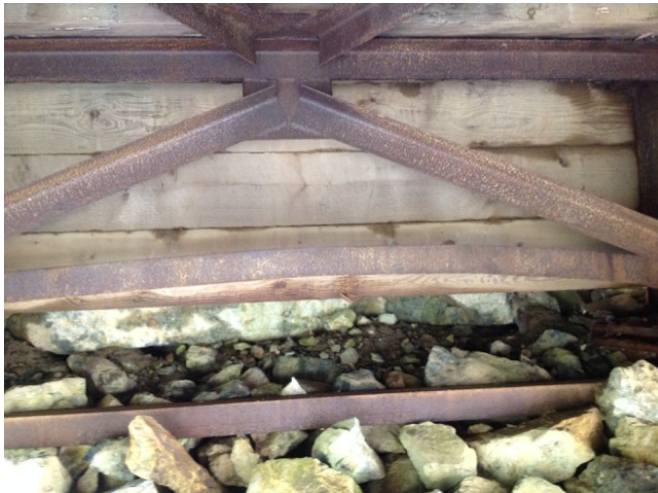
right abutment bottom cord on diaphragm
