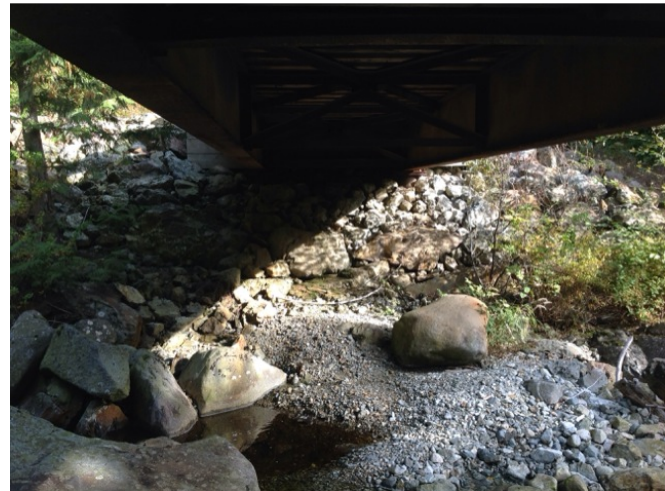
Left Bank Abutment when facing downstream
