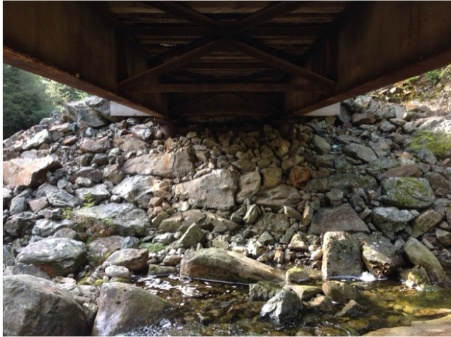
Right Bank Abutment when facing downstream
